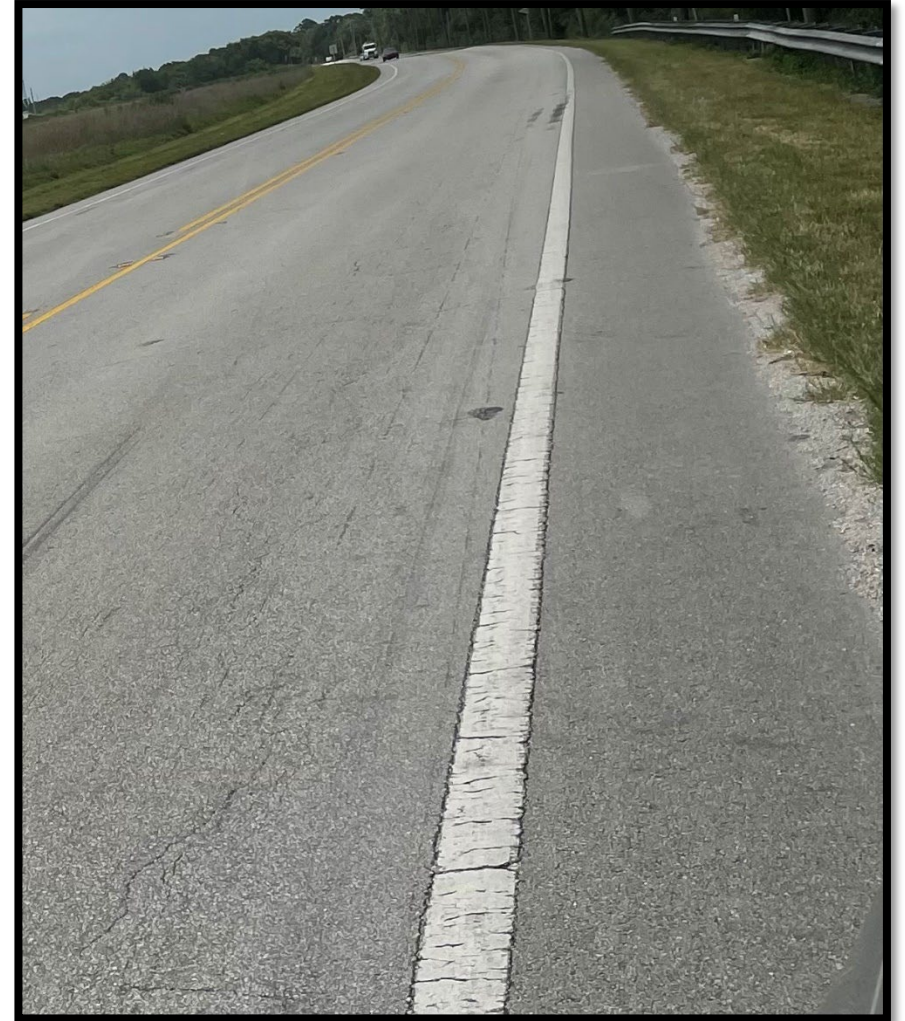
Northbound SR 19 US 98 (pre-construction)
