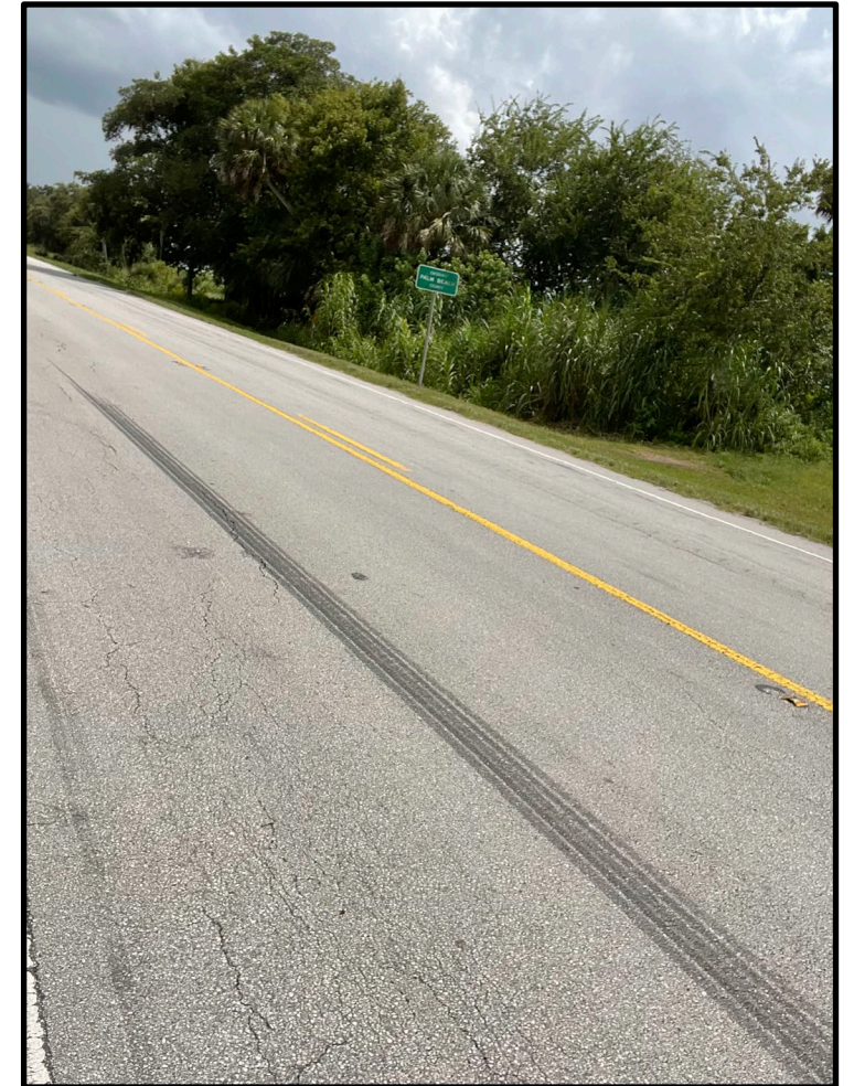
Southbound SR 19 US 98 (pre-construction)
