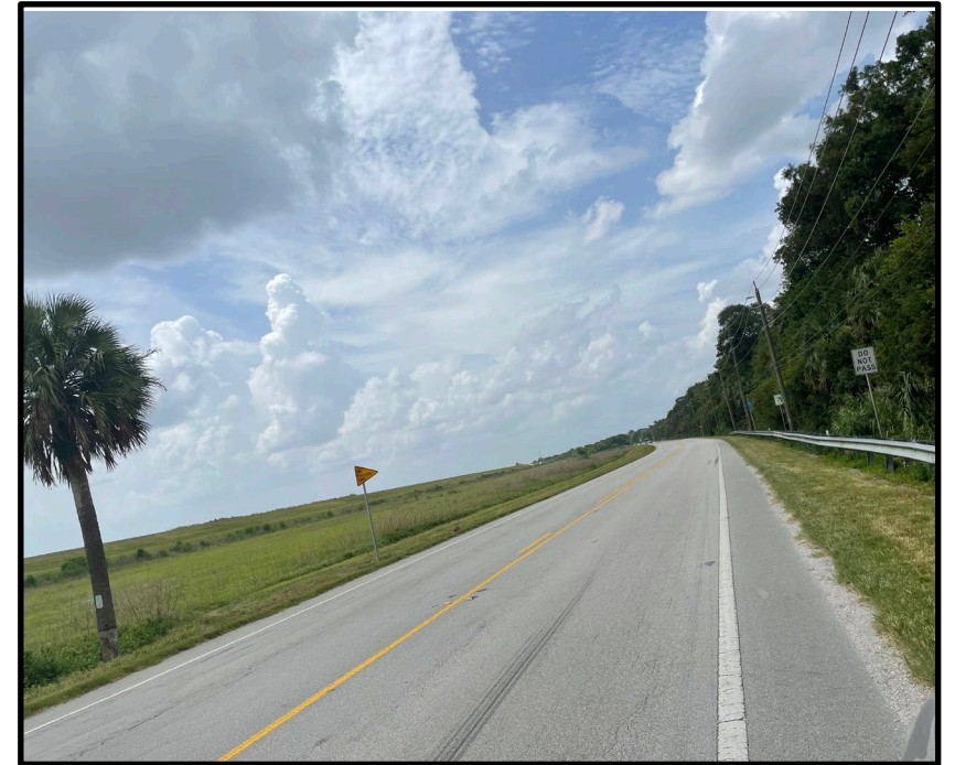
Northbound SR 15 US 98 (pre-construction)
