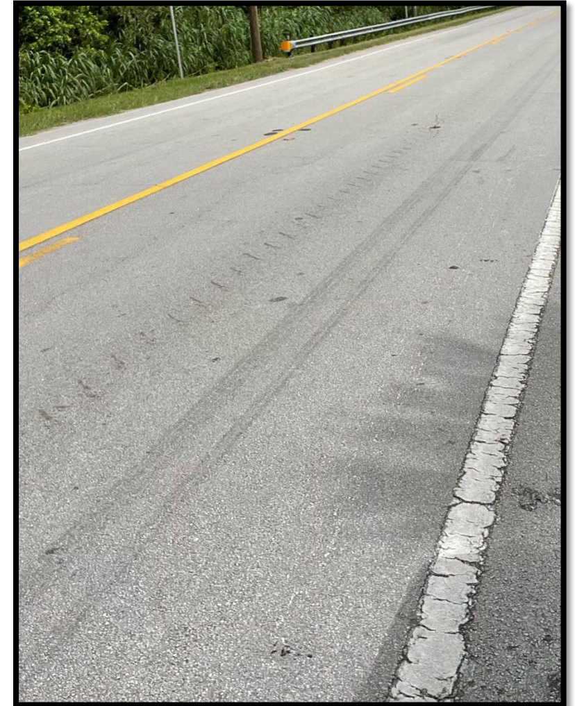
Southbound SR 19 US 98 (pre-construction)
